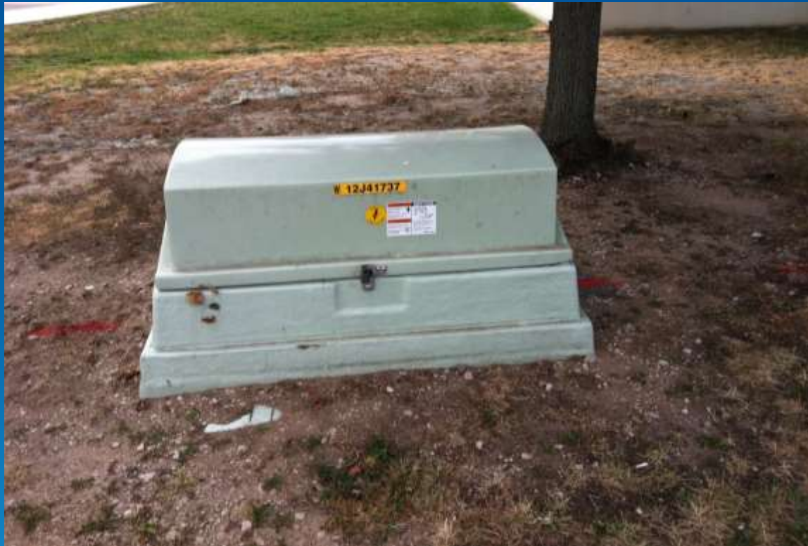
Above Ground Locking Fiberglass Enclosure
