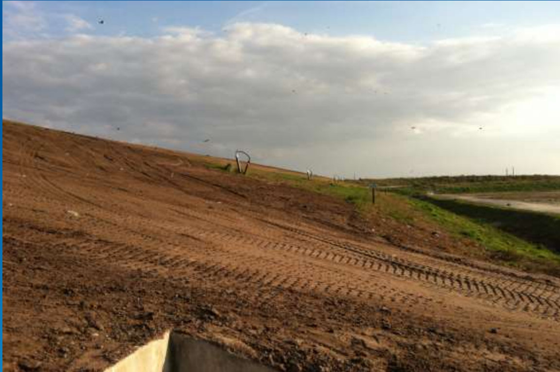
Typical Above Ground Wellheads
