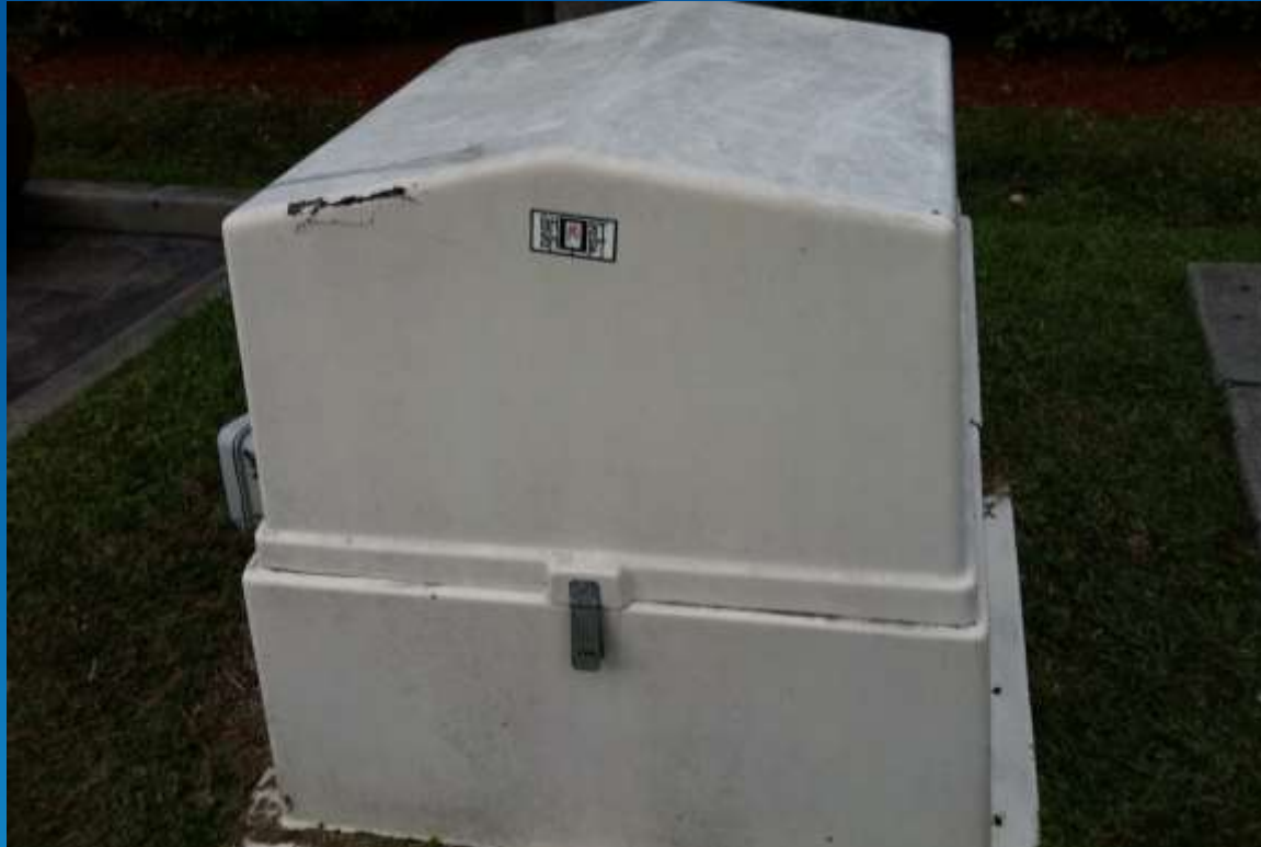
Above Ground Latched Fiberglass Enclosure
